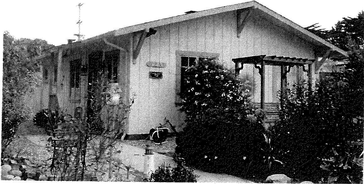
Photo #1. Looking south at the NE facing facade, & NW side-elevation. February, 2014.
